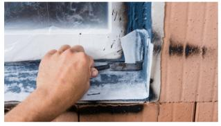
7. Install the AEROSANA FLEECE sub-sill flashing
