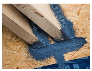
9. The finished joint at a double collar tie penetration
