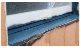
6. Pre-spray the sub-sill flashing
