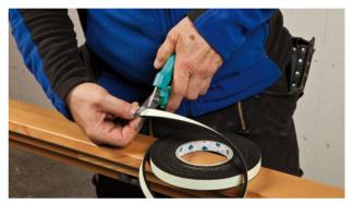
**4. Cut off the start of the tape** Roll off a length of CONTEGA FIDEN EXO and cut off the overcompressed start of the tape (approx. 2 cm (7/8")).
