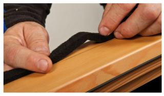
**6.** Allow for slack in the tape Allow for a small amount of slack in the tape when sticking it in place, particularly near joints – do not stretch the tape!
