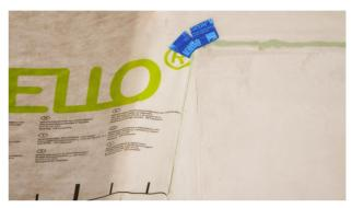
12b. Sealing to plastered chimney (insulated or double-shelled)
