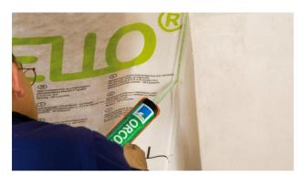
12a. Sealing to plastered chimney (insulated or double-shelled)
