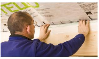
11b. Sealing to roughly sawn timber
