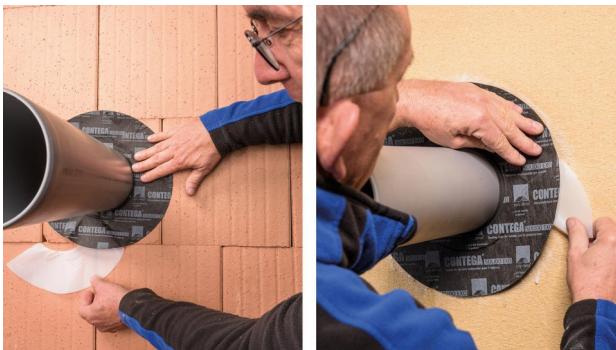
3. Stick to the subsurface Gradually remove the release film and stick the grommet to the subsurface with no folds or creases. Wood fibre should be treated with TESCON PRIMER.
