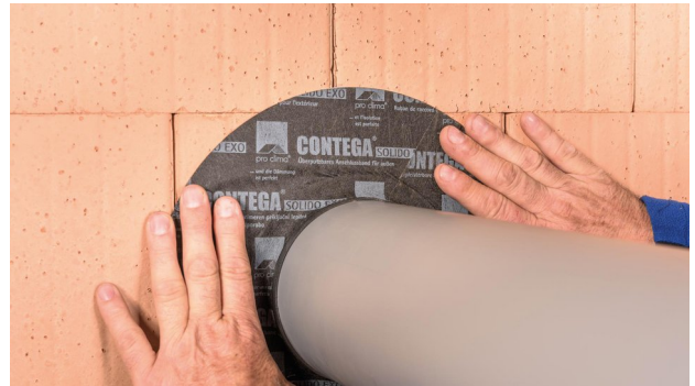
2. Position the grommet Hold the grommet at the EPDM sealing ring, slide it over the pipe using moderate force and position it on the wall.
