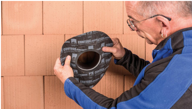
1. Pull the grommet over the pipe Pull the grommet over the open end of the pipe.
