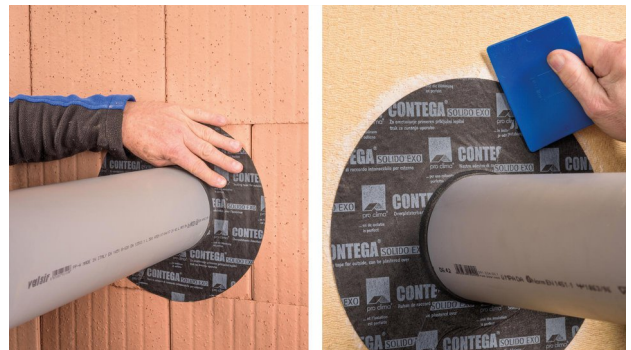
4. Rub in place Rub the adhesive bond evenly and firmly into place. This step can be carried out in a manner that is kinder to your hands by using the pro clima PRESSFIX application tool.
