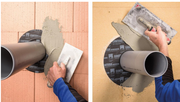
5. Plaster over the grommet Plaster over the entire surface of the grommet using suitable plastering systems.
