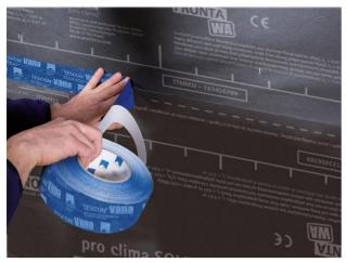
5a. Alternatively: Taping over the overlaps with TESCON VANA
