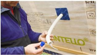
**1. Select suitable diameter** Select the size of the air-sealing plug to match the diameter of the conduit.
