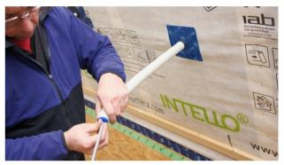
**4. Create an airtight bond with the conduit** Push the plug firmly into the conduit as far as it will go.
