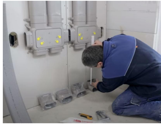
Watch our video on how to clean the install ComfoTube Flat 51 ductwork.
